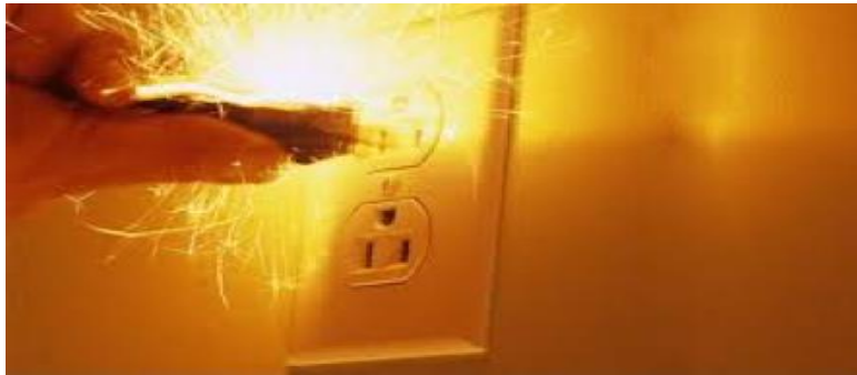
Figure 2. Arc causing fire on the socket
